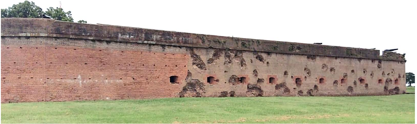
The corner of Fort Pulaski where the breach occurred was rebuilt without embrasures for lower tier cannon.
